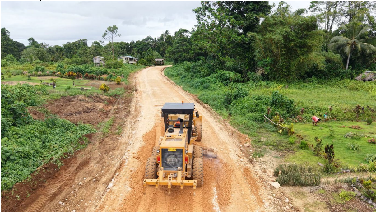
Photo 2 - Road rehabilitation works underway on the East Road as part of the Australia–Solomon Islands partnership to improve national transport connectivity.
