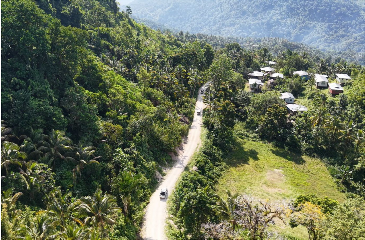
Photo 1 – The upgraded Busurata Road has reconnected communities to markets, schools and essential services across central Malaita.
