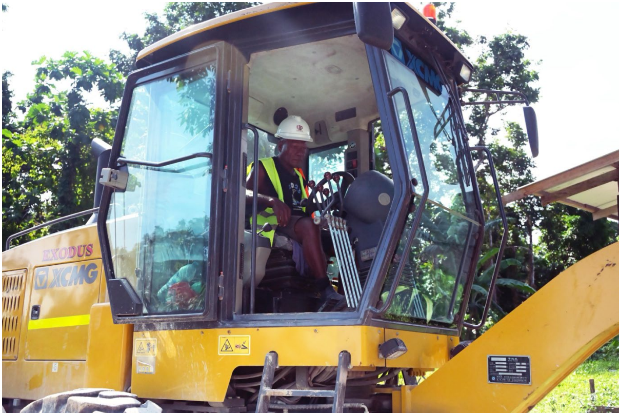
Photo 6 – The 11 projects across Honiara and Malaita have all been delivered 100 per cent by Solomon Islands workers.
